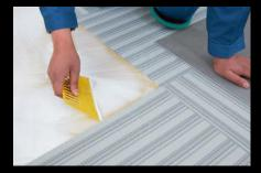
**O5.** After installation, use a roller to crosswise roll over each piece of woven flooring, so as to ensure elimination of the air under the woven flooring and tight bonding between the woven flooring and the floor.
