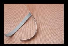
**O4.** If chemical splicing is adopted, masking tape should be first used at during splicing; apply pressure to tape with a hand or roller in order to firmly fix the tape. Then, use a rotating cutter or wallpaper cutter to cut open the tape at the joint; use special splicing glue, and insert the needle head into the woven flooring joint; move the glue tube along the joint; 10 minutes later, carefully tear off the tape along the reverse direction.
